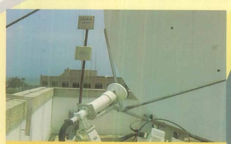
Figure 6: Two BWA antennas at 3.5 GHz can be clearly seen just close to receiver front
